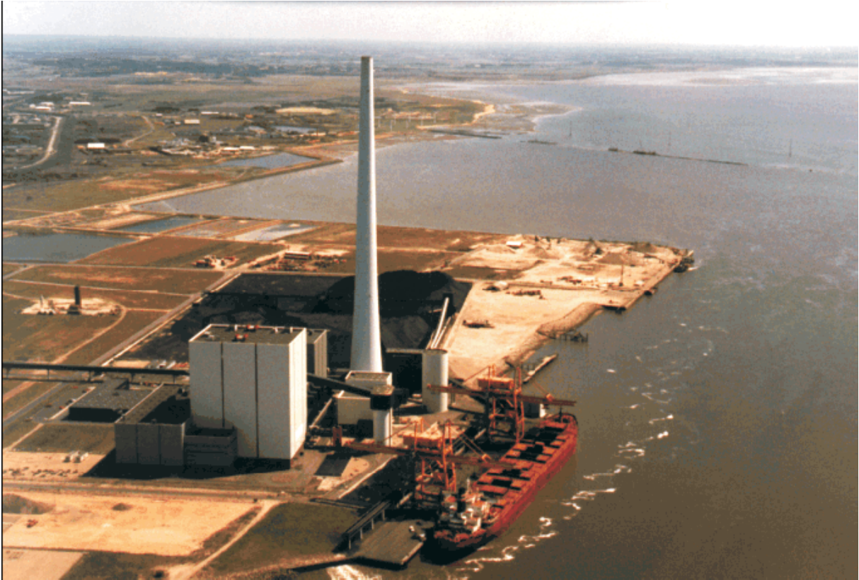
Figure 1: A modern coal fired power station [2]
